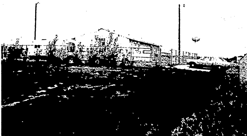
Figure B-43. Indian Health Center, Shonto. View Looking North.
